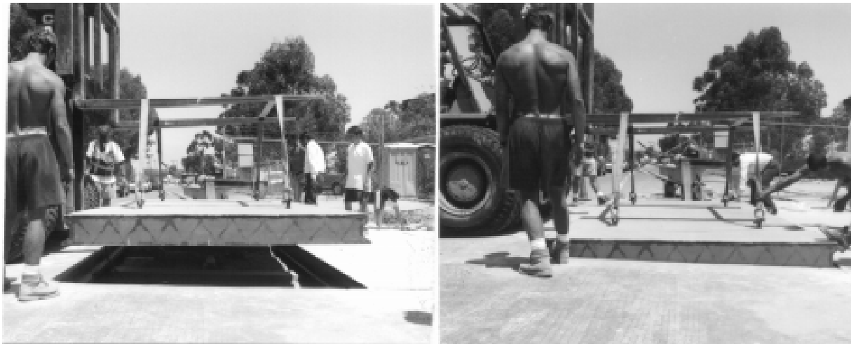
Fig. 10: Stages in the Placement of Composite Decks in a Road Test-Site
