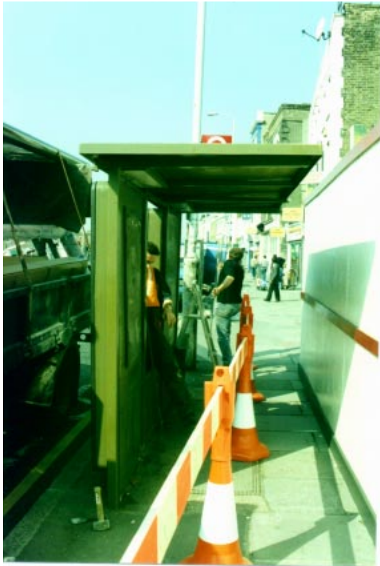
Fig. 2: Photograph of the bus shelter prior to its removal
