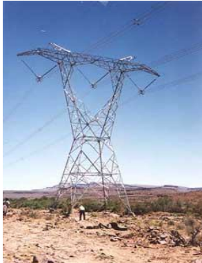
Fig.1. High voltage transmission lines.
